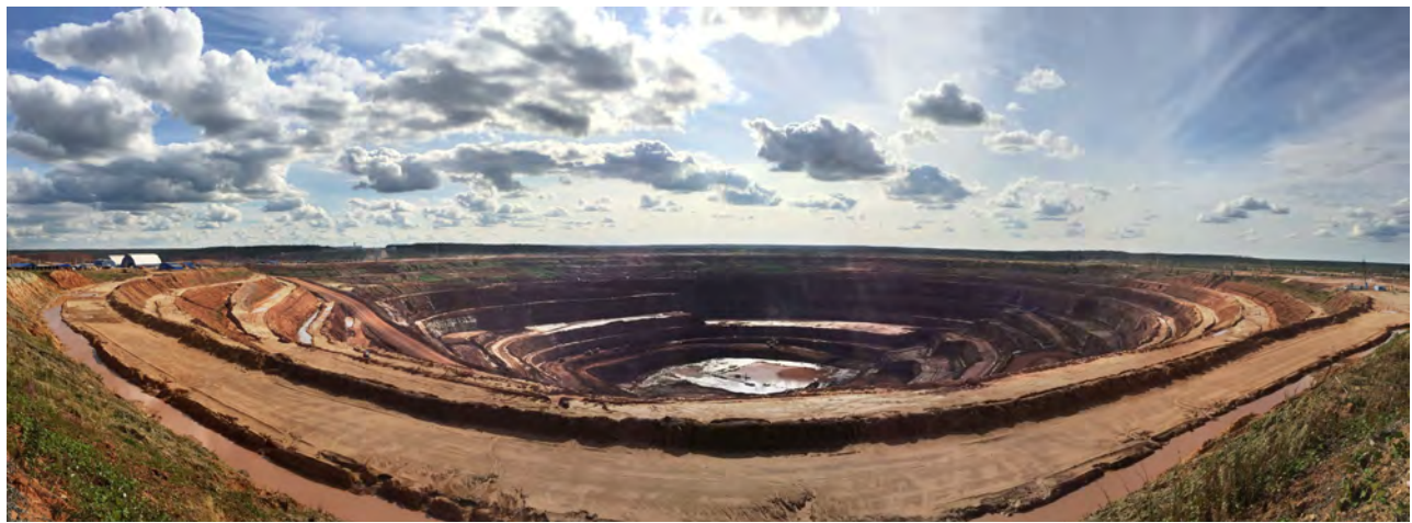
Figure 10. Open pit of the Arkhangelskaya kimberlite in August 2016, which at the time spanned 1.1 km. Arkhangelskaya was the first of the six kimberlites at Lomonosov to be developed since it had the least overburden and the largest diamond reserve. Photo by Karen Smit.
