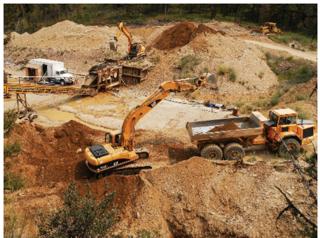
Figure 44. Excavators and a washing plant on Gem Mountain process gravel for sapphire recovery. Photo by Warren Boyd.
