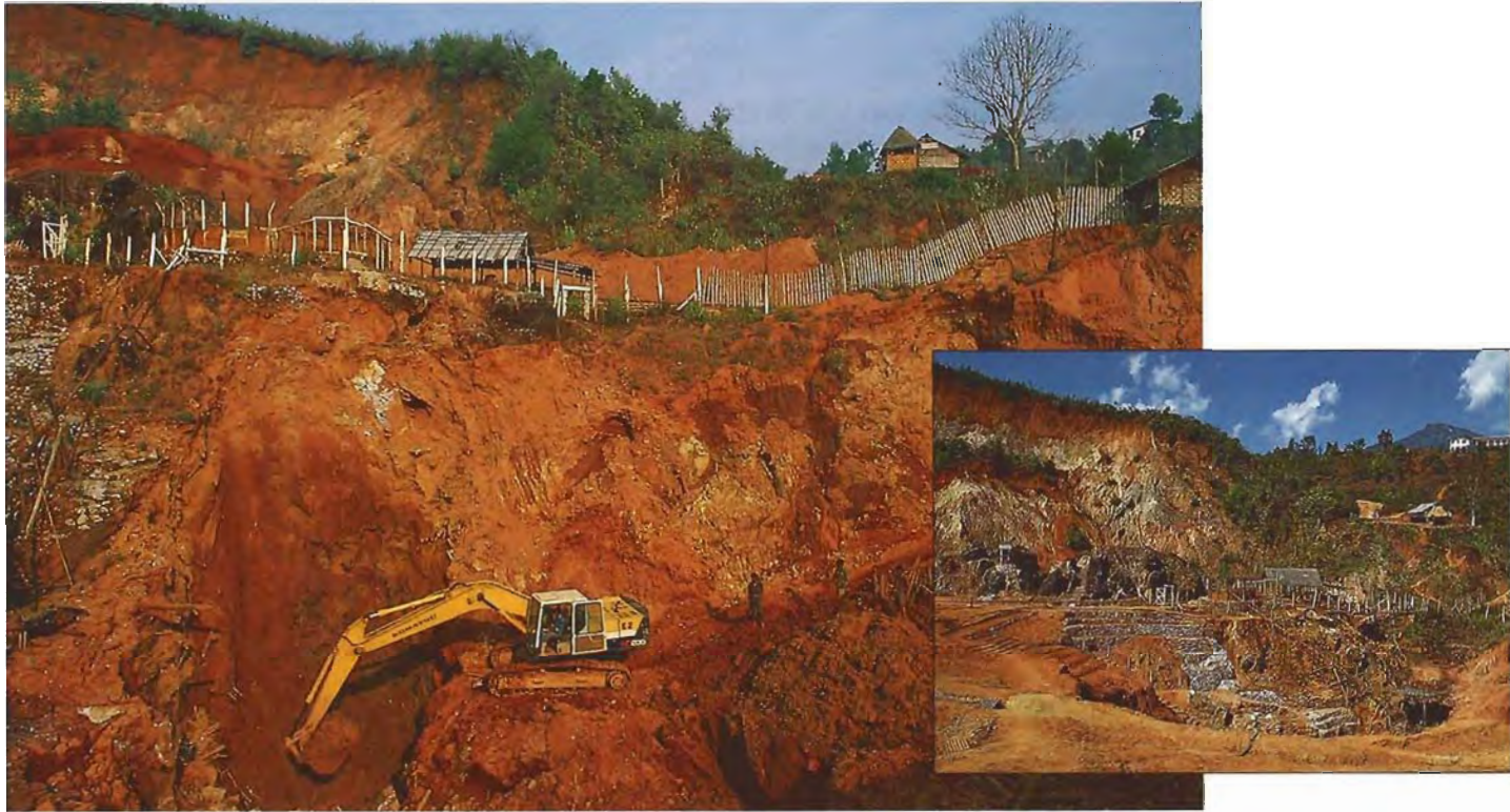
Figure 13. In 1991, the MGE open-pit mine at Shwe Pyi Aye was being worked by hand (inset); through the use of heavy earth-moving equipment, many tons of overburden had been removed by the time of the 1992 visit (main photo). The backhoe shown was removing byon, which was subsequently taken by truck to the Central Washing Plant. Photo by Robert E. Kane.
